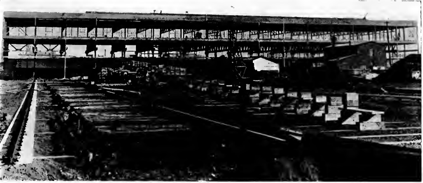
The new ship ways and the new ship tool shed of the Pusey and Jones plant.
